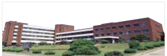
SK Chemicals R & D Center
