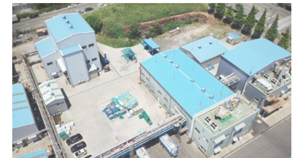
Under construction of a PO3G facility
